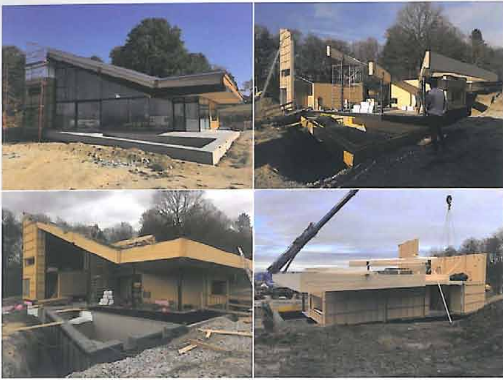
建築結構施作過程 THE PROCESS OF BUILDING CONSTRUCTION
